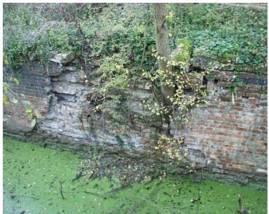
The lock is surrounded by trees of various ages and sizes. Many are elms which have dutch elm disease and are dead or dying. There are perhaps half a dozen larger trees growing on, or out of, the structure including a particularly large one growing on the top sill and another at the bottom of the the lock.
