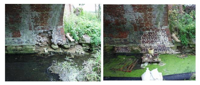
Working on the lower parts of the structure is difficult due to the presence of rubble, silt and water bot upstream and downstream of the bridge. Water flows down the canal for much of the year so it is not possible to simply dam off each side of the bridge and pump out the middle except potentially during long dry periods in the summer.
